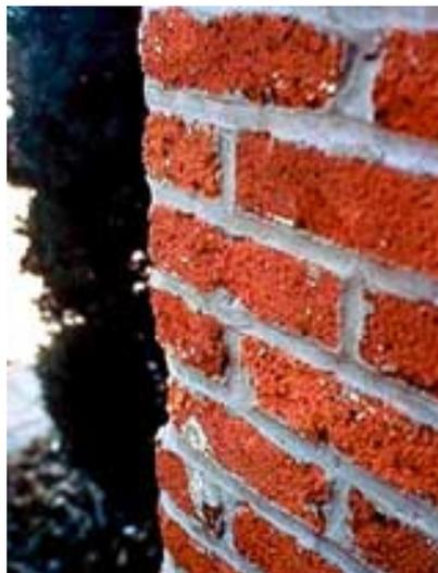
Sandblasting can remove the protective outer layer of brick allowing it to absorb moisture and quickly deteriorate.
